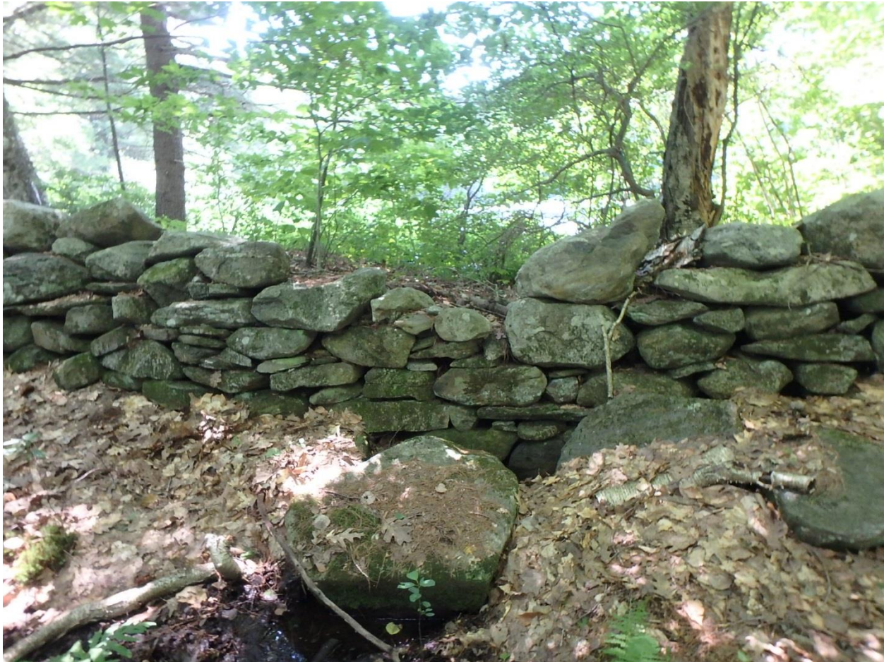
Figure 2.17 – View of Auxiliary Dike
