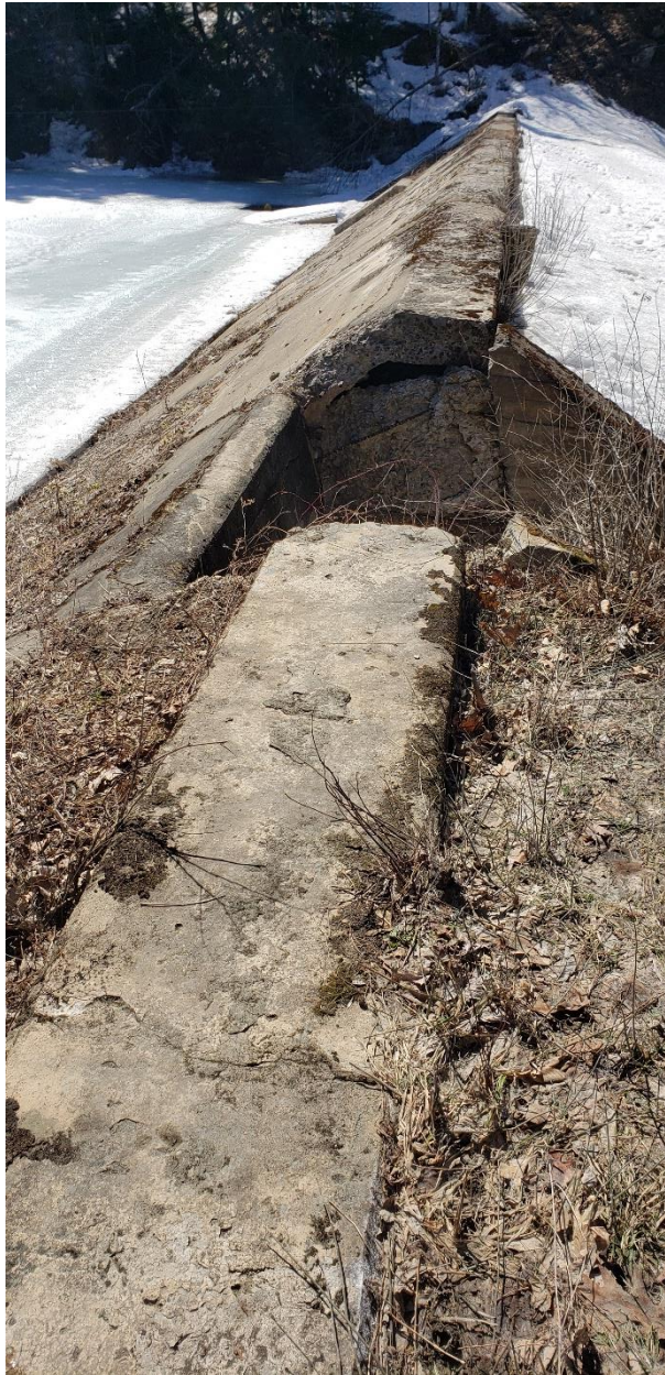
Figure 2.15 – View of Dam and Spillway from Right Abutment
