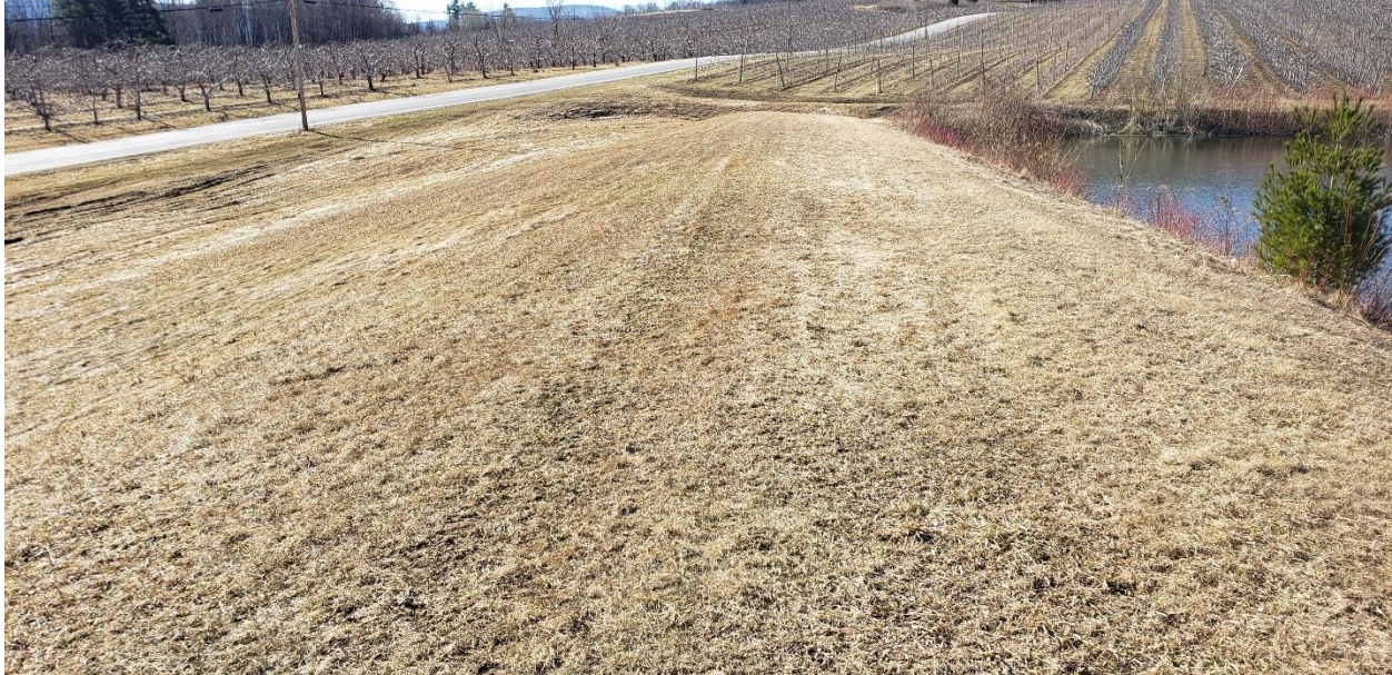
Figure 2.18 – View of Dam and Spillway from Left Abutment
