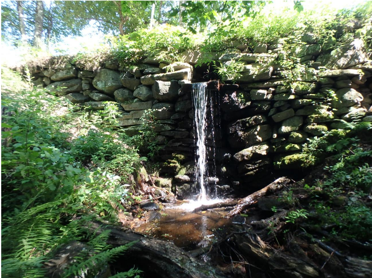
Figure 2.16 – View of Dam and Spillway from Downstream Side
