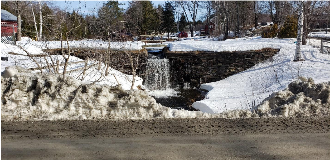
Figure 2.14 – View of Dam and Spillway from Downstream Side
