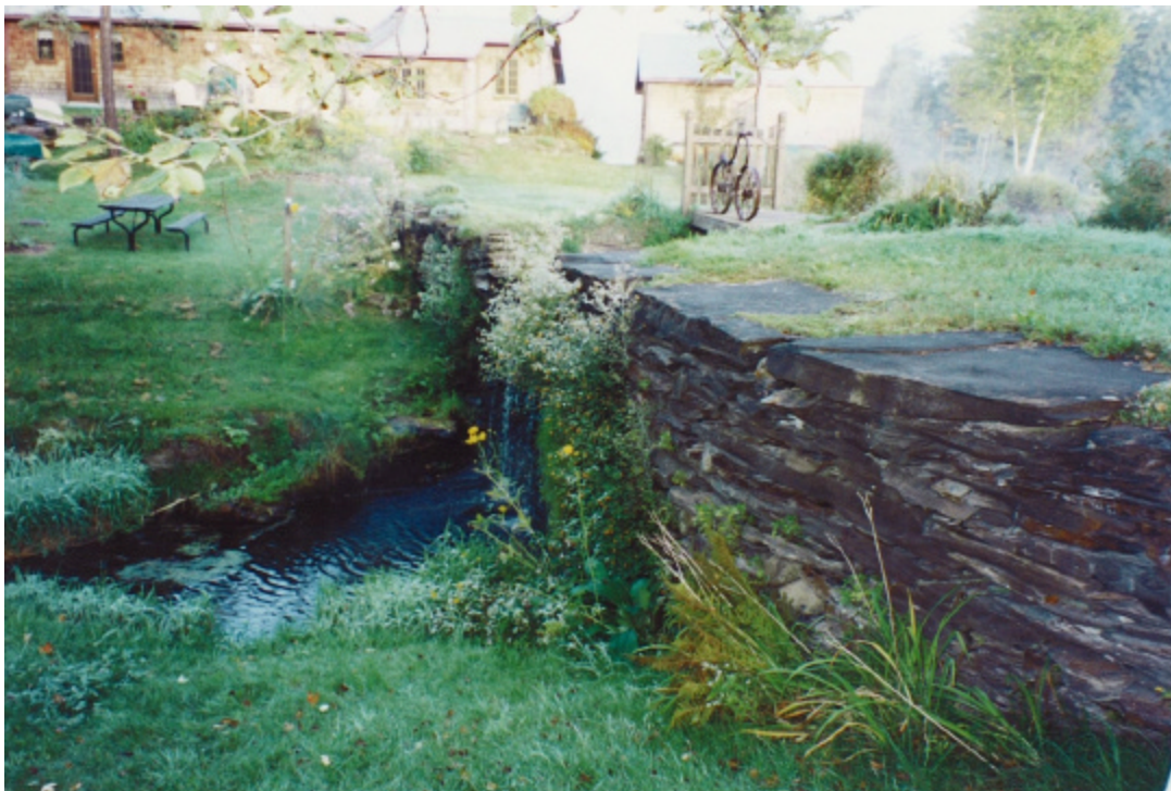
View looking along the dam. Note the slight lean of the downstream face.
