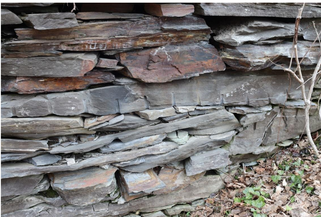
Figure 21. Closeup view of downstream stone masonry wall of the Curtis Pond Dam showing several stones bearing plug and feather quarry marks.
