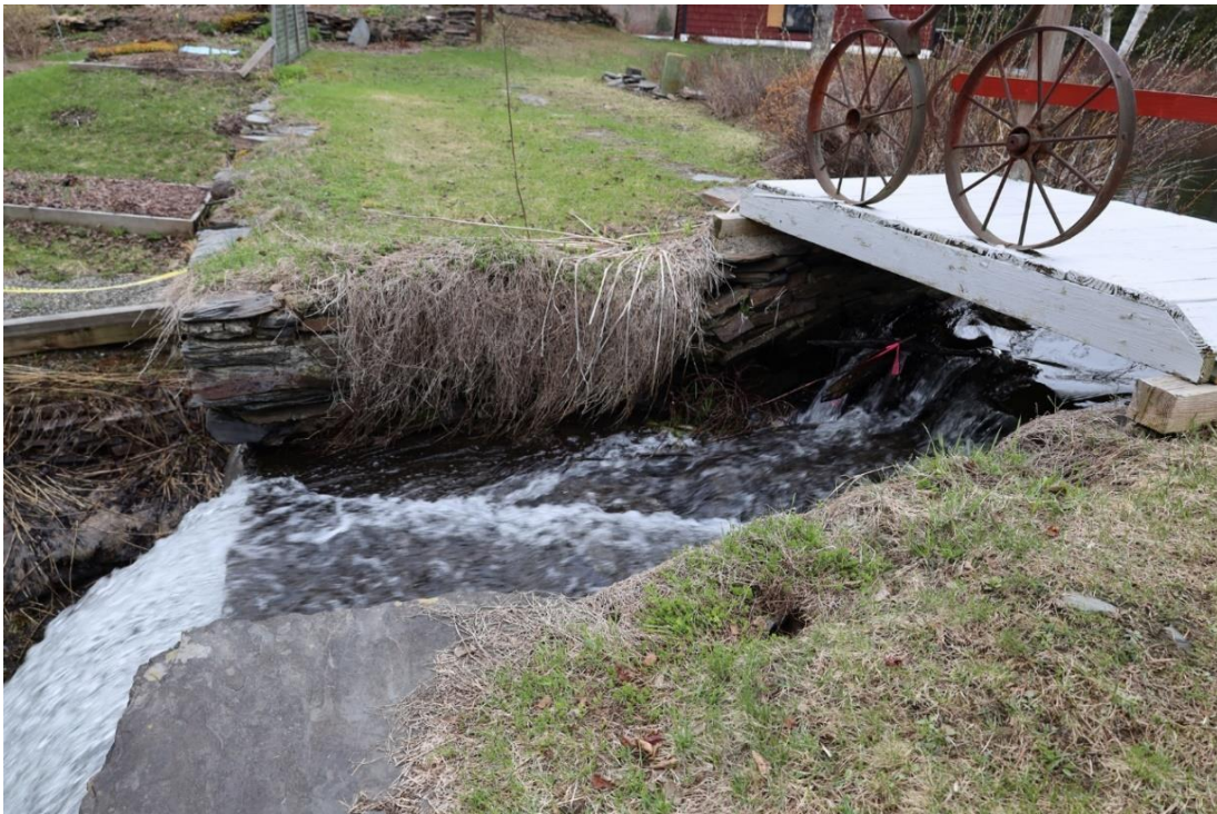
Figure 25. View northwest of the primary spillway of the Curtis Pond Dam; note stone lining sidewall within spillway.
