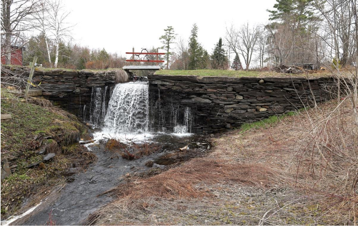
Figure 26. View north of the Curtis Pond Dam; note location of the low outlet structure, to the right of the primary spillway (approximate center of image).
