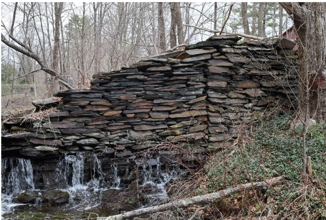
Figure 40. View north of the downstream side of the Maple Corner Dam showing a large construction joint, possibly marking the division between a foundation (right) and the dam (left).
