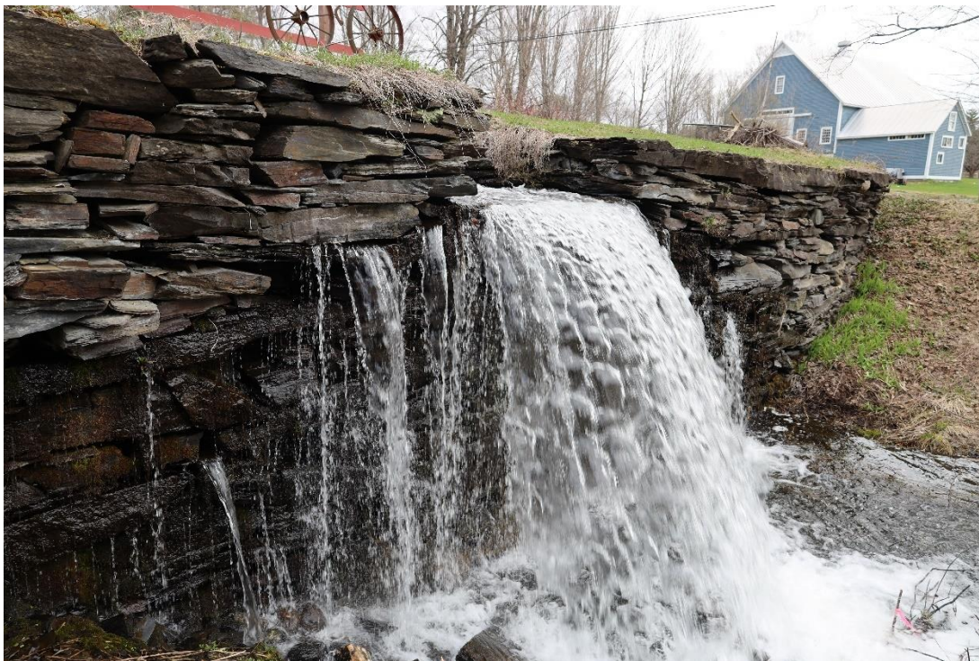
Figure 20. View east of downstream stone masonry wall of the Curtis Pond Dam showing unfinished quarried stone used in the construction.
