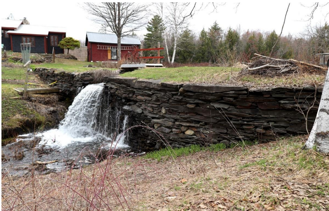
Figure 27. View northwest of the Curtis Pond Dam showing the curve of its left-hand side.
